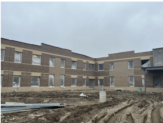
South Side Veneer Progress
