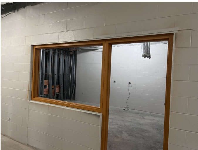
B-204 Corridor-Frames Painted, Walls Primed
