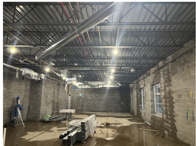
Music Room Progress
