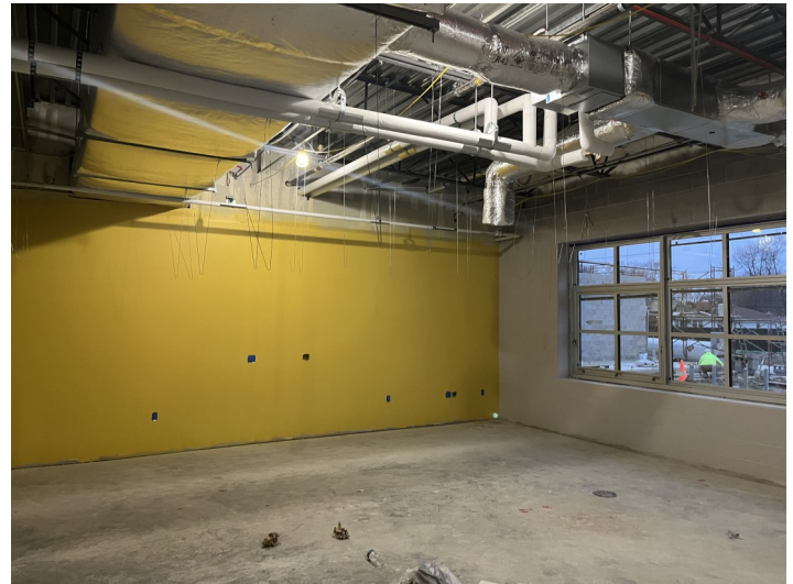
North End Classroom Progress
